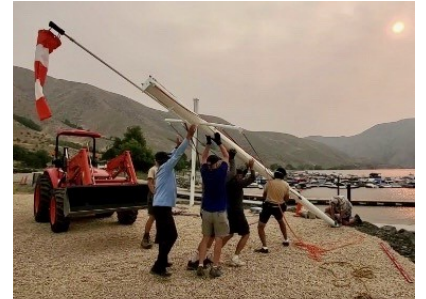
Installation of yardarm with windsock
